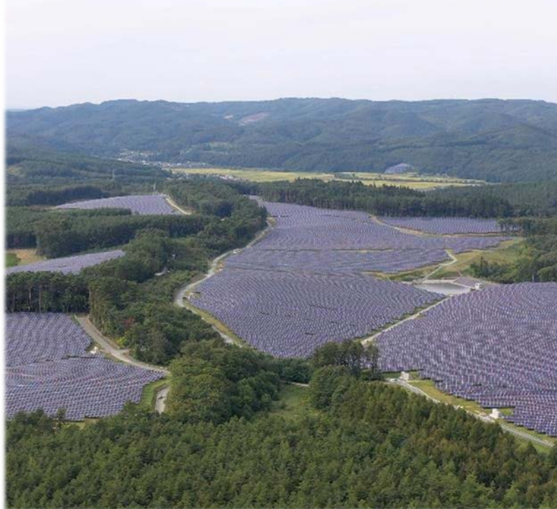
View of site (As of October 2021)
